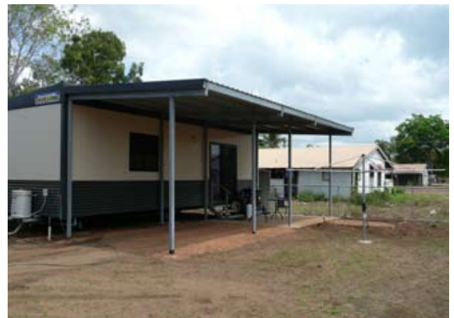
New 1 bedroom Staff Quarters
