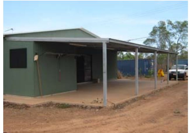
New 4 bedroom staff accommodation
