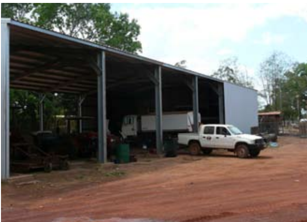
The New Shed
